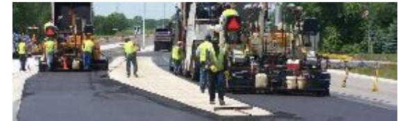
Warm Mix Asphalt
