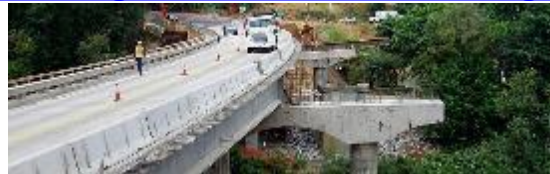
Prefabricated Bridge Elements and Systems
