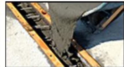
Ultra-High Performance Concrete Connections
