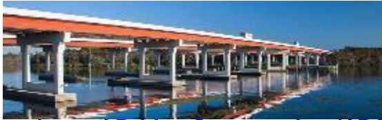
Accelerated Bridge Construction (ABC)
