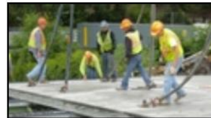
Ultra-High Performance Concrete Connections
